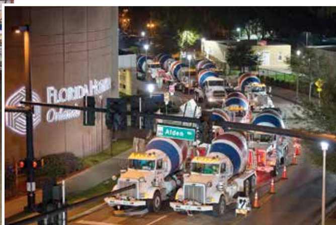
Work begins on the Florida Hospital for Women. Roughly 700 truck loads poured about 180,000 cubic feet of concrete into the slab.
