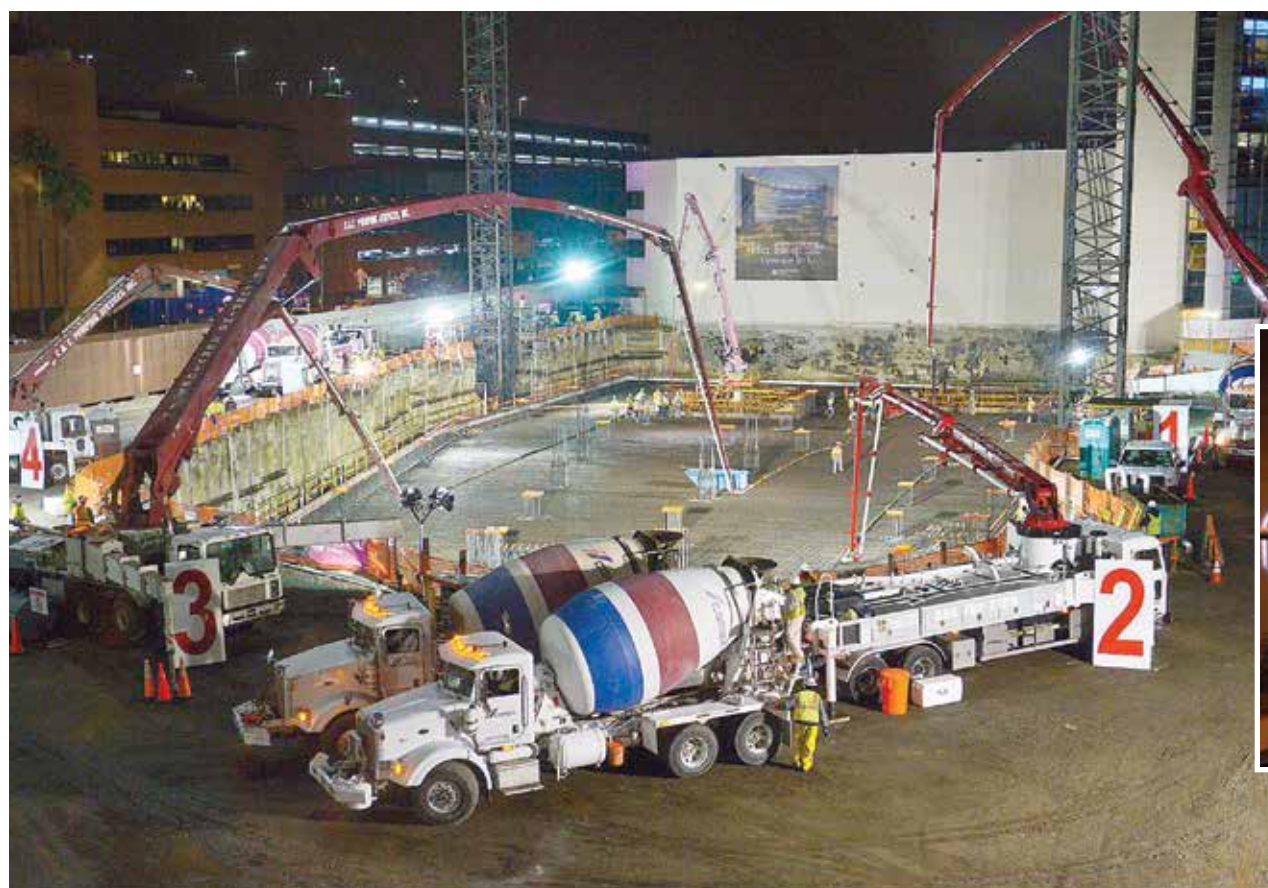
Work begins on the Florida Hospital for Women. Roughly 700 truck loads poured about 180,000 cubic feet of concrete into the slab.
